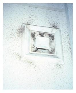
Third, the speed of the supply air across the ceiling thins the laminar boundary layer of air between the ceiling surface and the supply air. In areas 1-12 inches from the diffuser, the boundary layer thins enough to allow the mixture of particles from the room air and supply air to deposit at higher rates than at other surface areas in the room.
