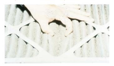
Make sure filters do not become overloaded and that there is no air bypass in the filter rack.
