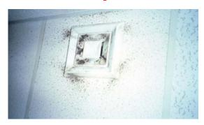
This is NOT an indication of a need to clean ducts rather, an indication of a lot of particles in the room air which deposit quickly near the diffuser because of the boundary layer effects caused by the jet of air at the diffuser.
