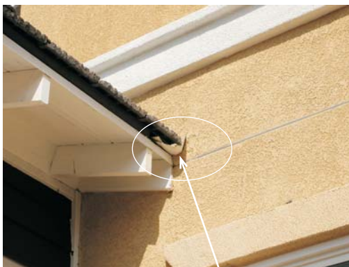
Kickout Flashing , which keeps water out of the vertical adjoining wall
