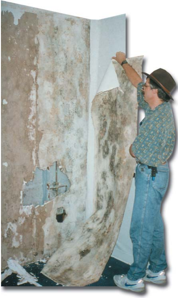
Fig. 1 Mold in new construction
