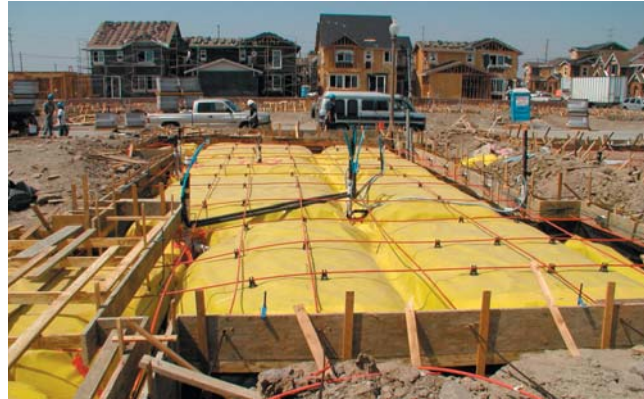
Fig. 3.8 Installing the vapor retarder and capillary break layer is difficult under slabs with grade beams
