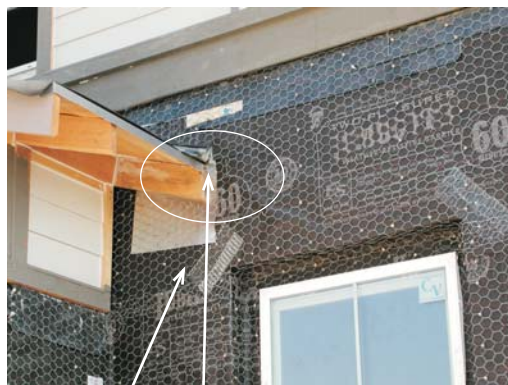
Kickout Flashing , which keeps water out of the vertical adjoining wall
