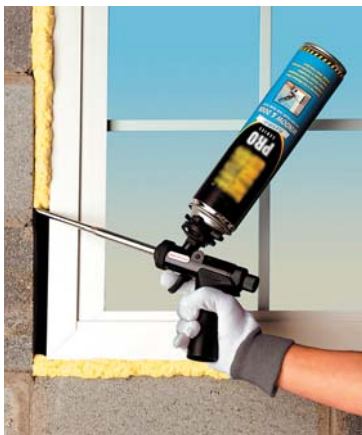
Fig. 3.12 Air seals help exclude wind-riven water
