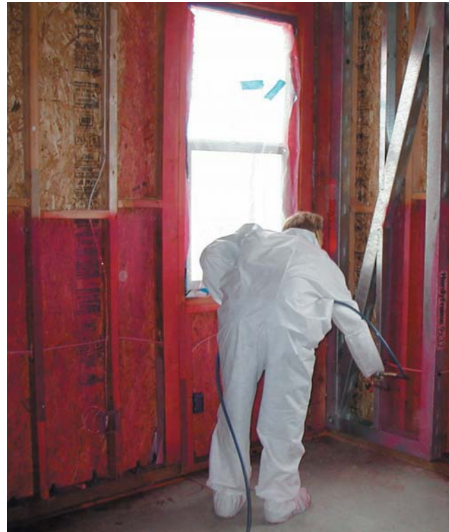
Fig. 4.9 Mold-resistant sealers can extend safe drying time
