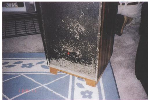
Concealed mold growth on the back of a stereo speaker against an exterior wall.
