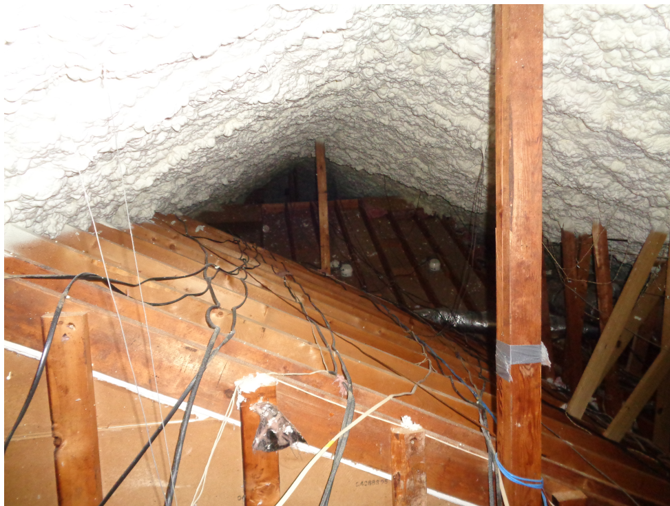
Figure 1. Photograph of polyurethane spray foam (SPF) with high chemical emissions applied to underside of a roof.
